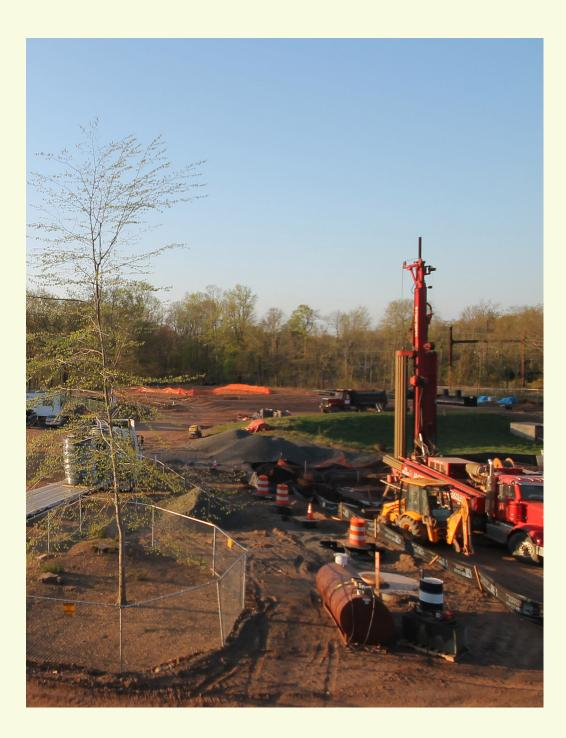
Left: Drilling of a test geothermal borehole on campus.
